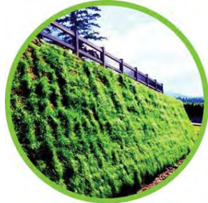
Vegetated Retaining Wall
