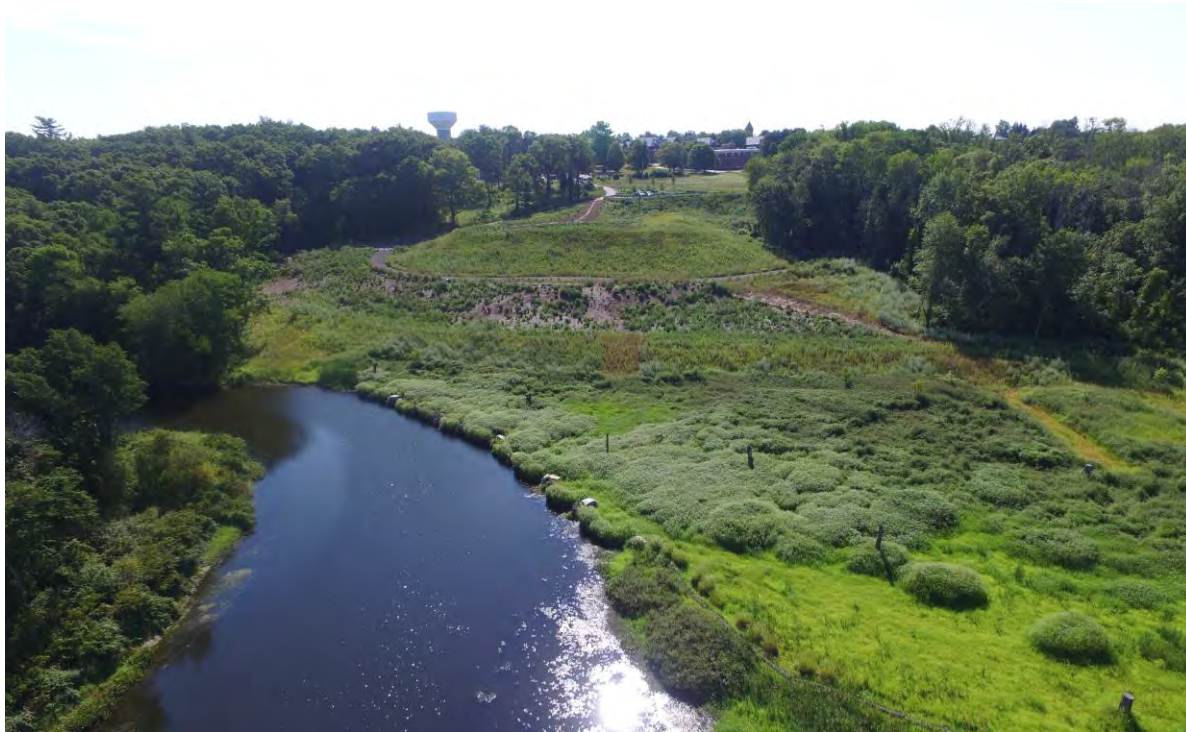
Medfield State Hospital, Remediation along the Charles River
